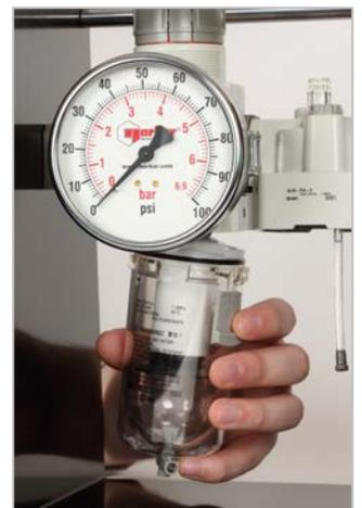
**FIGURE 7 – Replacing the Filter Element**
